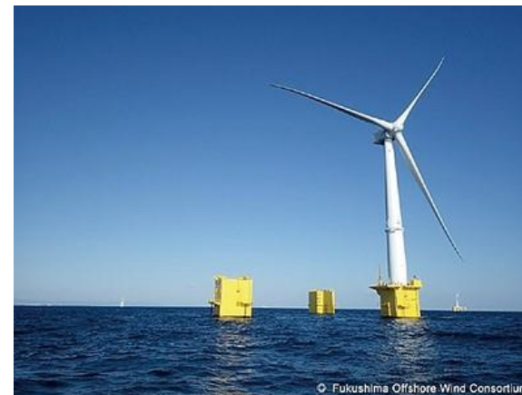
7 MW Semi-Sub Photo Credit: Fukushima FORWARD
